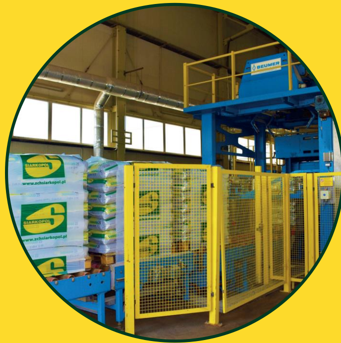
Reconstruction of the product packing and dispatch system
