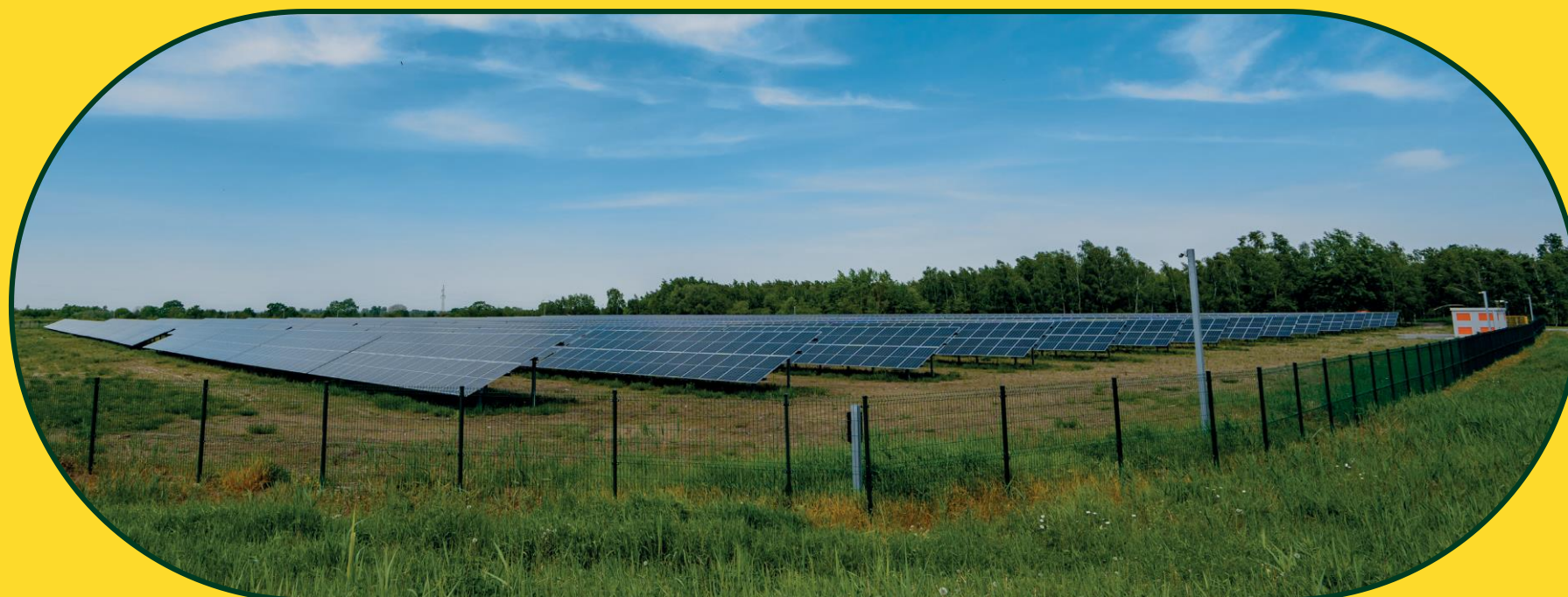
Launch of a 2 MW photovoltaic farm supplying electricity to the Company
