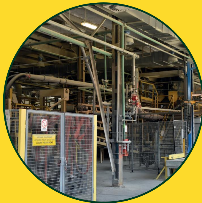
Construction of a second packing and palletizing line
