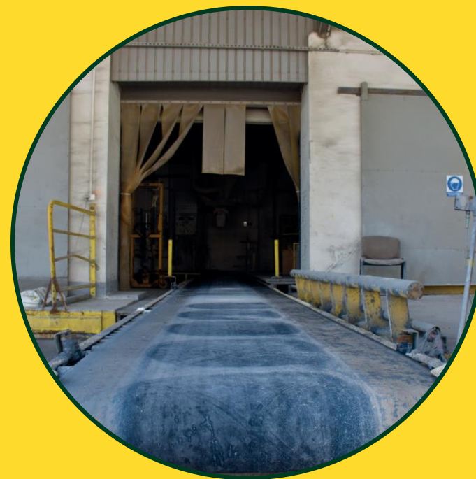
Modernization of exhaust gas treatment systems for granulated fertilizer production.
